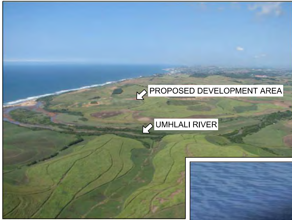
1 LOOKING SOUTH FROM THE TINLEY MANOR NORTH BANKS
